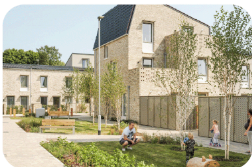
New energy efficient housing scheme in Norwich, source: Mikhail Riches Architects
